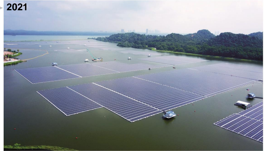
60MWp Tengeh Floating Solar Farm
